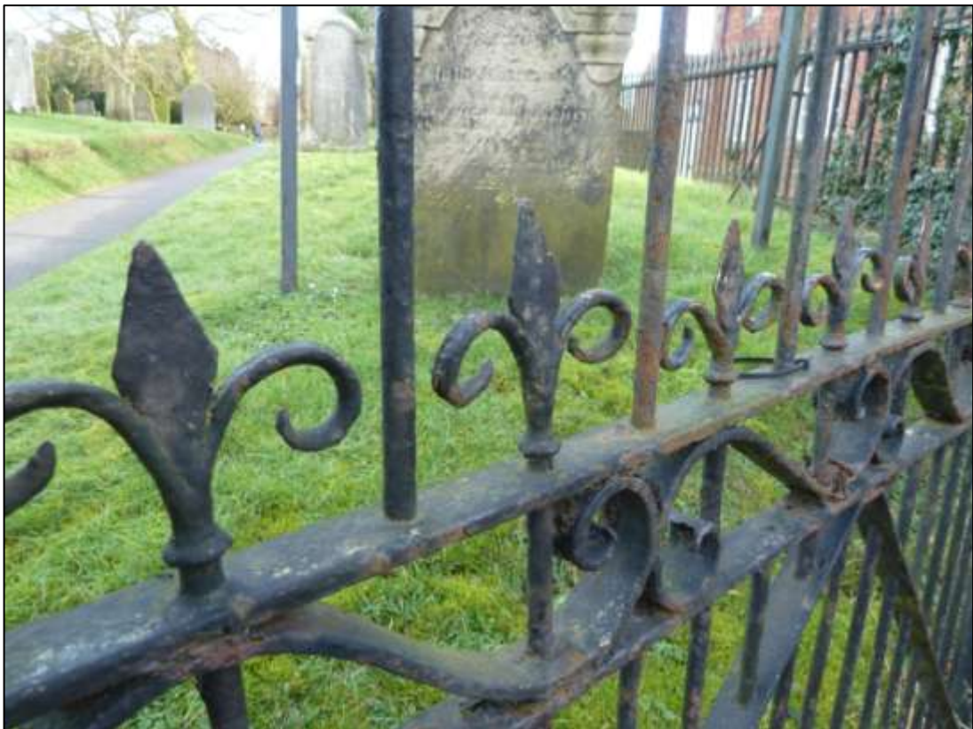
Figure 19 Wrought iron railings at the south entrance to the churchyard
