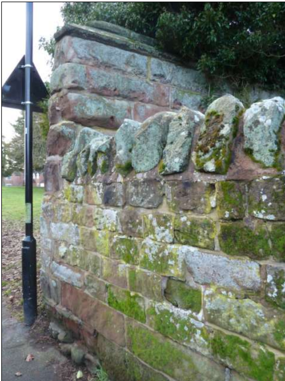
Figure 20 Church boundary wall and truncated boundary wall formerly stretching to Parkside
