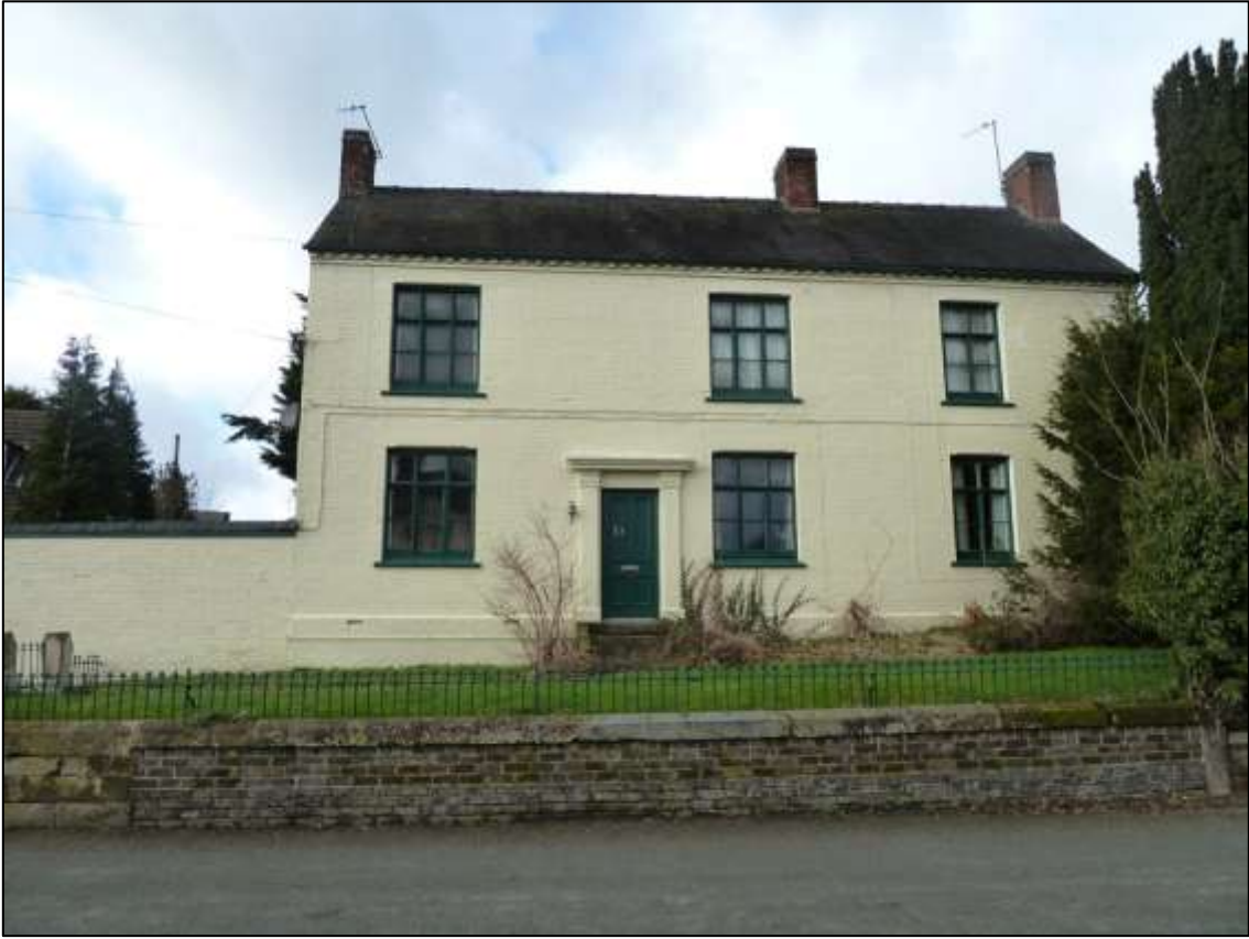
Figure 43 Properties at the northwest of the conservation area
