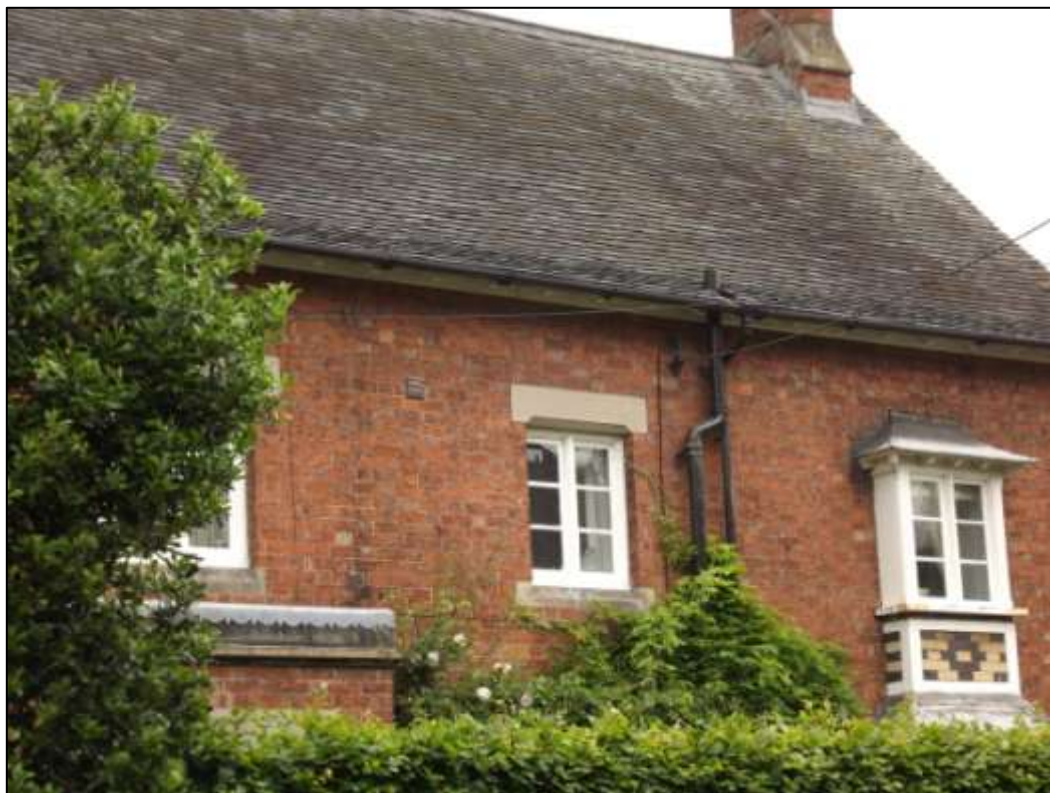
Figure 10 Church House with two storey, square set bay windows
