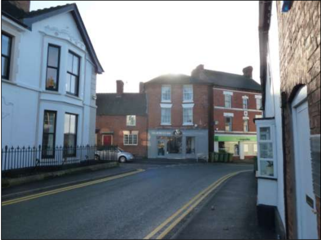
Figure 23 The contrasting heights and ages of buildings along High Street add variety and create interesting views.
