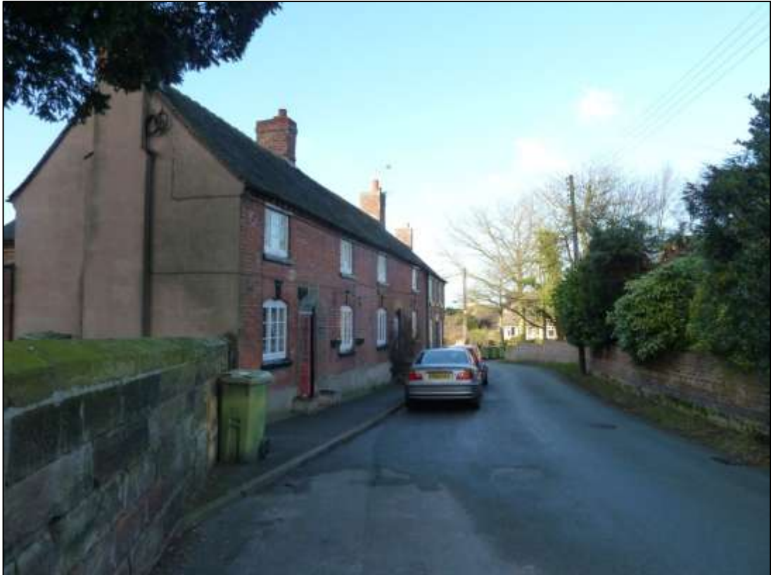
Figure 8 Casements at 3 Sellman Street
