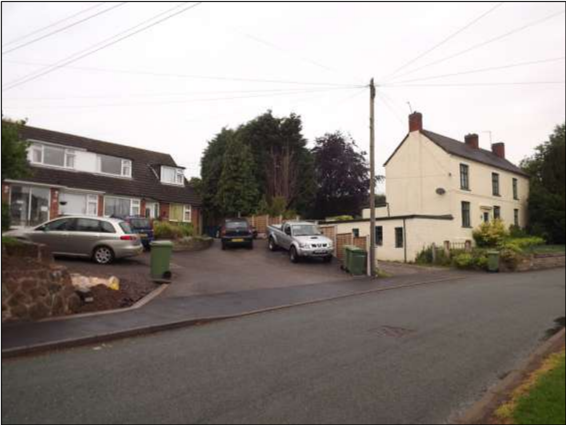
Figure 42 Properties at the northwest of the conservation area
