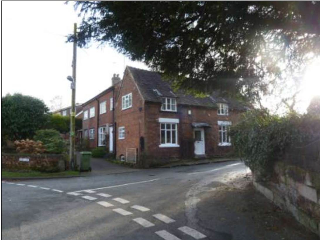
Figure 6 St Lawrence Cottage. The main façade of this cottage faces the church. Historic paving is visible in front of the cottage.
